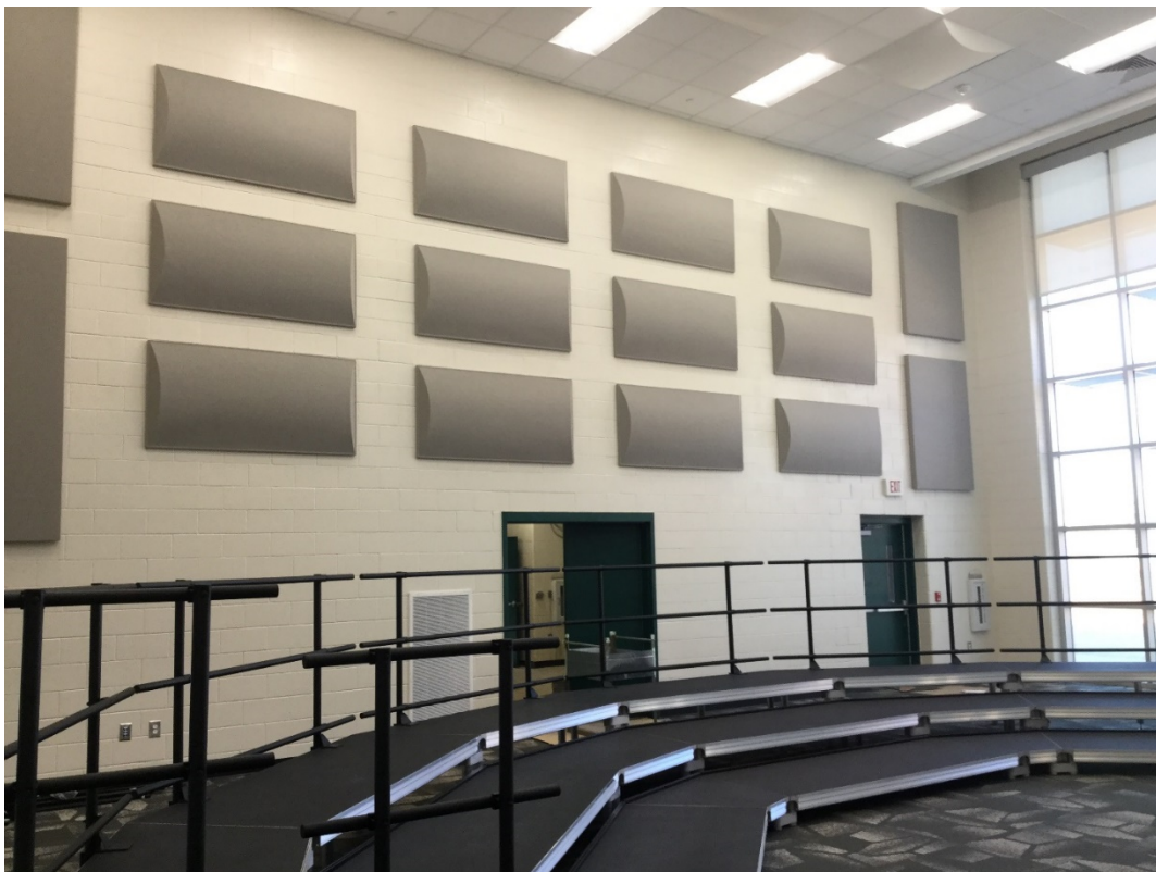
Chorus room stands and acoustical finishes complete.
