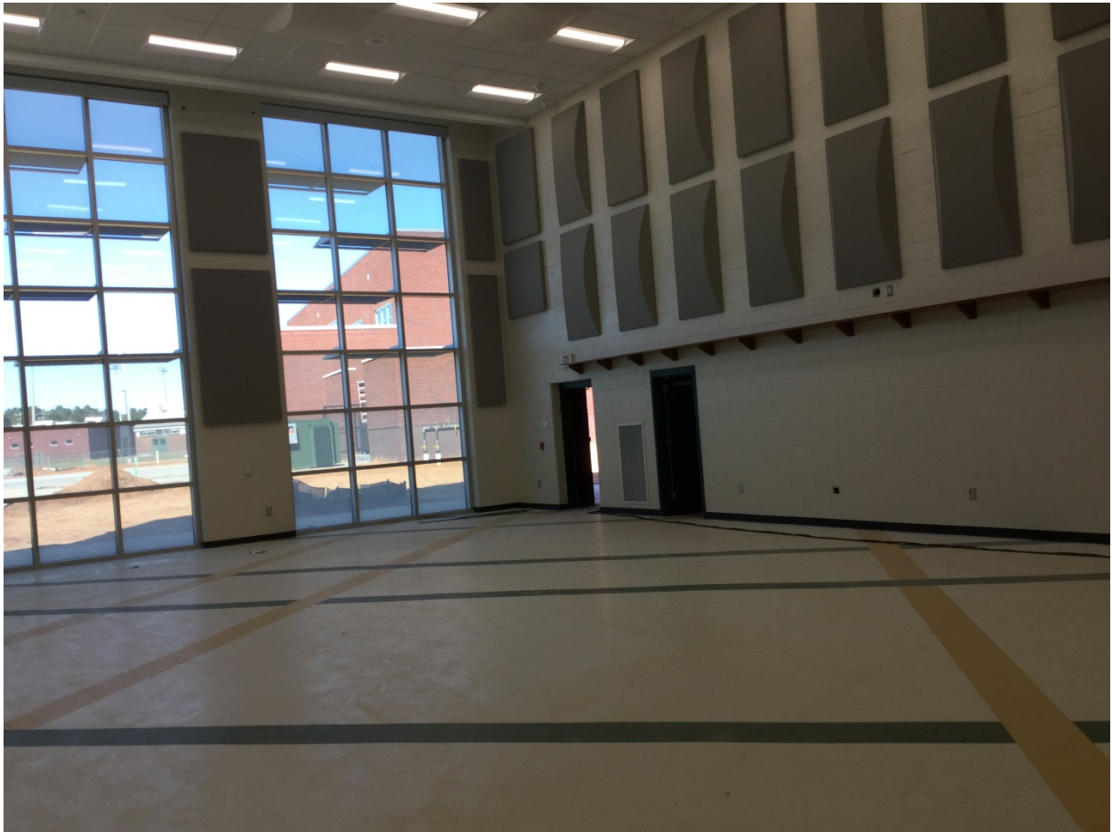
Finishes complete in Band Room.
