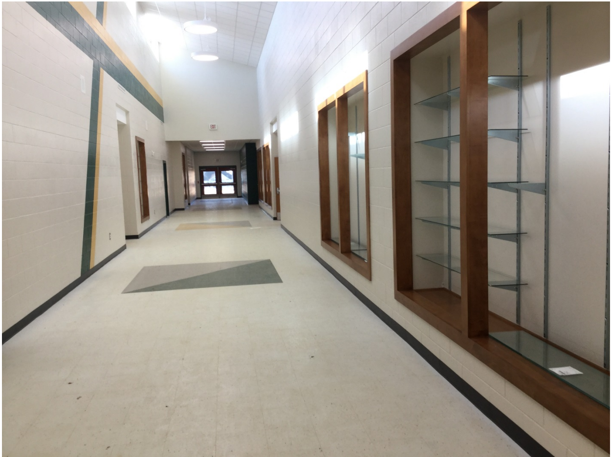
ROTC/Band Building display cases in corridor complete. Ready for final cleaning and waxing.
