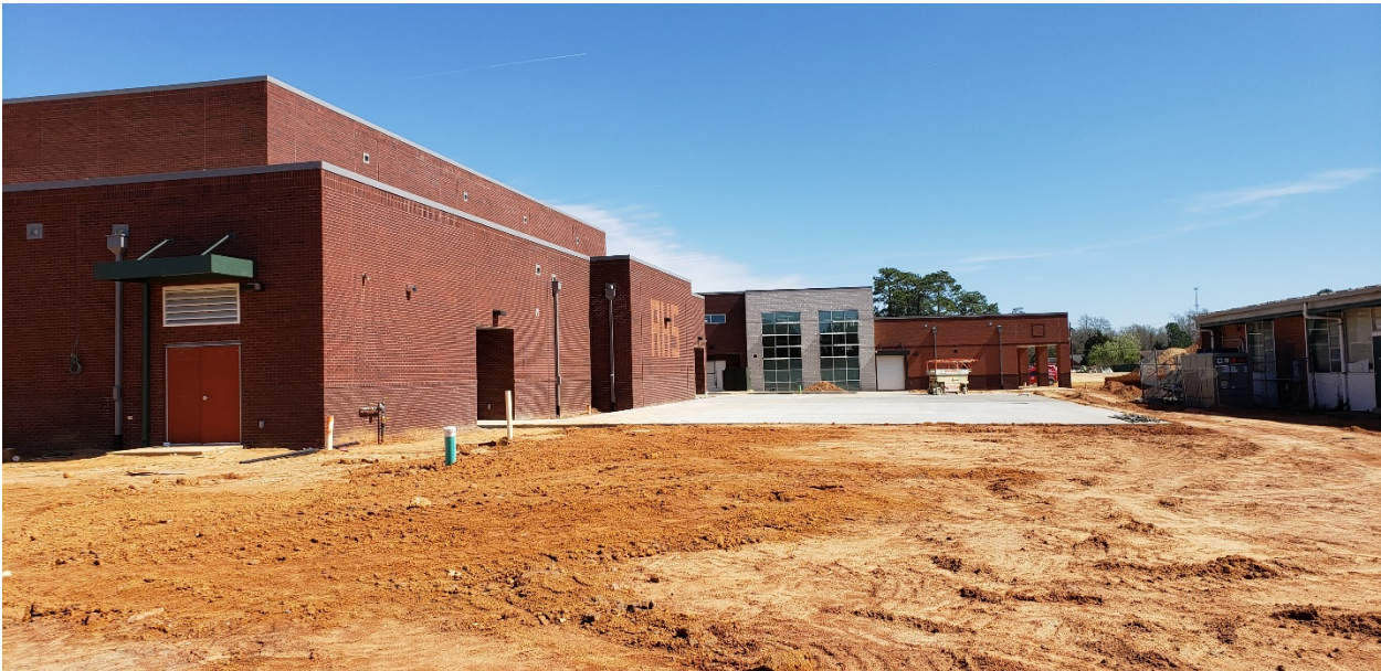
Final Grading and backfill of sidewalks underway.
