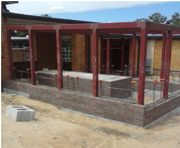
Gloverville - Steel and Masonry
