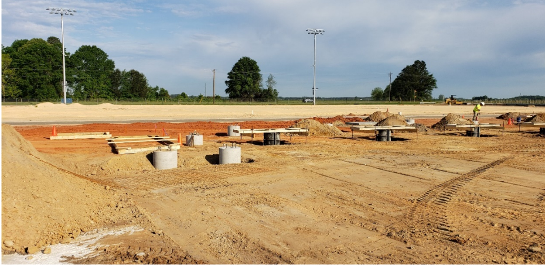
Football field – bleacher/press-box foundations
