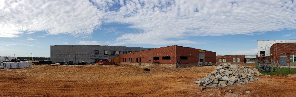
Area "A" – Classroom Exterior
