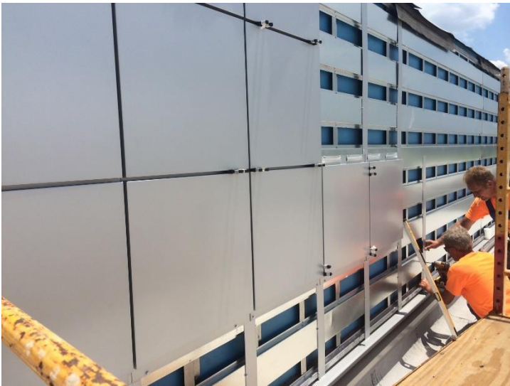
Metal wall panels in selected areas being installed
