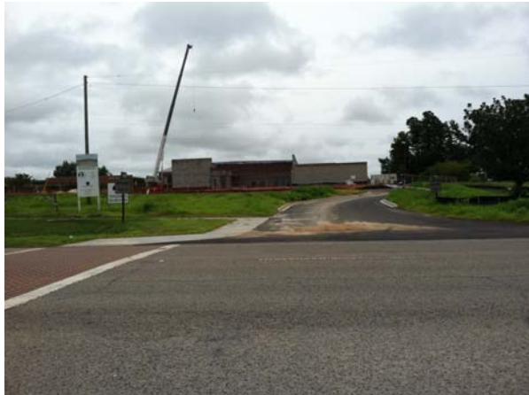
1 – Addition viewed from Atomic Road. Crane is placing steel framing for the roof.
