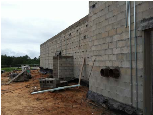
3 - Exterior walls at mechanical room and kitchen.
