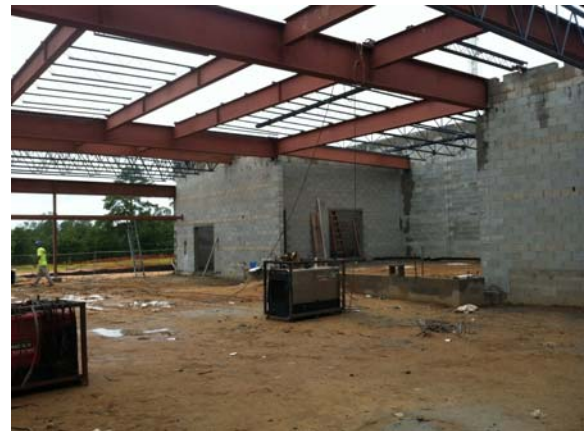
2 – Dining Room. Stage to the right, window wall to the south.
