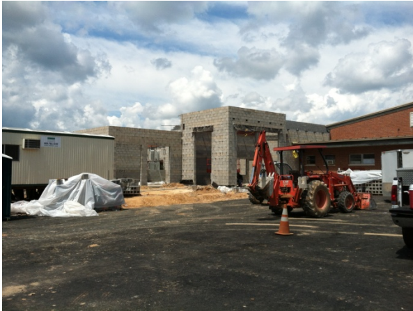
1 – Concrete masonry walls at the north entrance and kitchen are complete.
