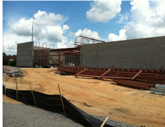
2 – Addition facing Atomic Road. Large opening in the center is for the dining room. Roof steel is ready to set.
