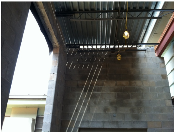
3 - Roof joists and deck over the connecting corridor adjacent to the existing gymnasium.
