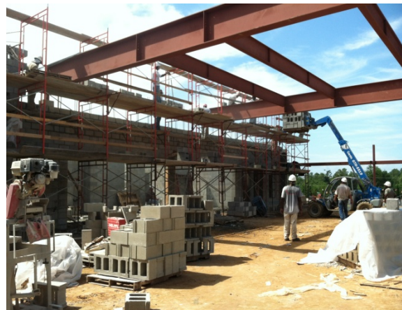
4 - View of new dining room. Masons are at work on wall above kitchen serving line.
