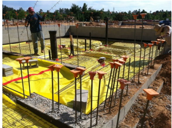
2– Boys and Girls toilet rooms. Note yellow vapor barrier installation. CMU wall cavities will be cleared of debris.
