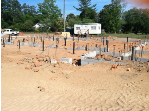
1 – Kitchen area viewed from Dining Room. Note plumbing stub-ups from under slab roughed-in waste plumbing.
