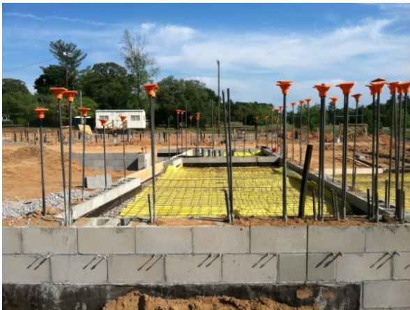
3- Stage Storage Room. Stage floor is elevated, cafeteria table and chair storage room is to the right.
