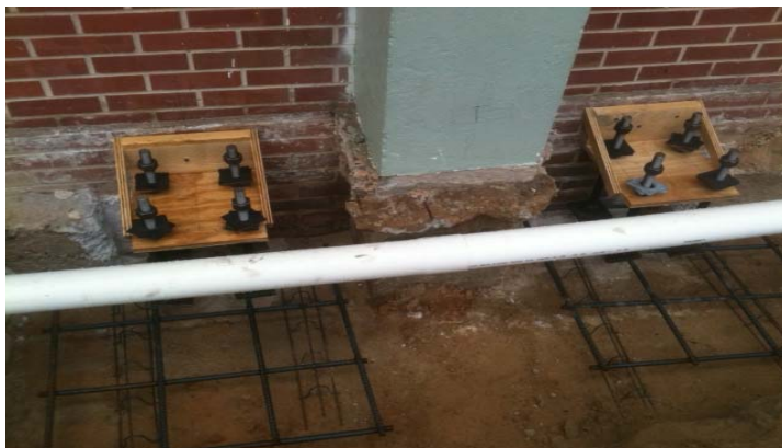
1 Rebar and anchor bolts for column footings at gym.
