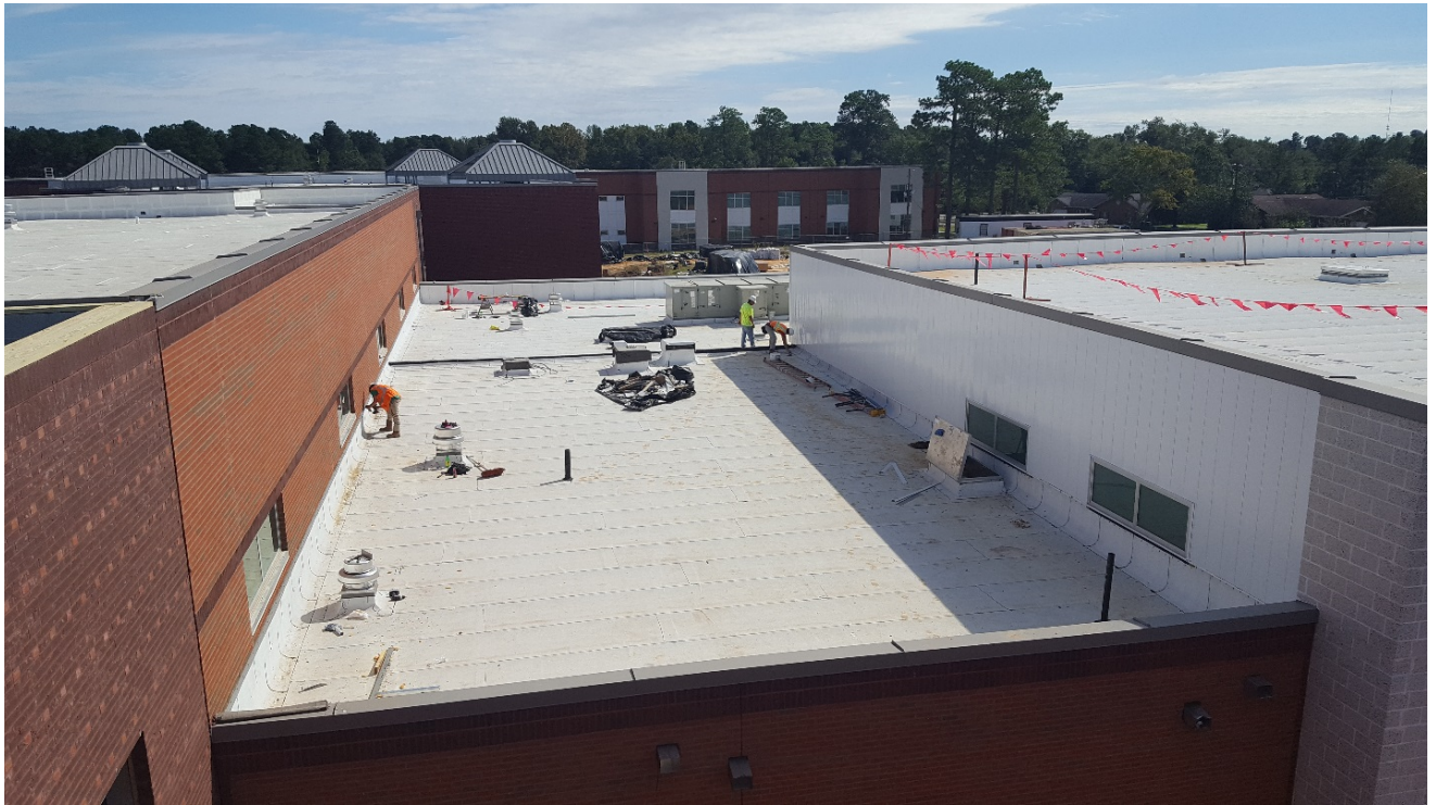
Roofing and metal wall panels at the ROTC Band Building.
