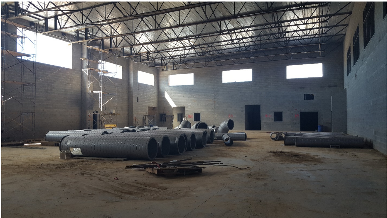
Ductwork started in Gym.
