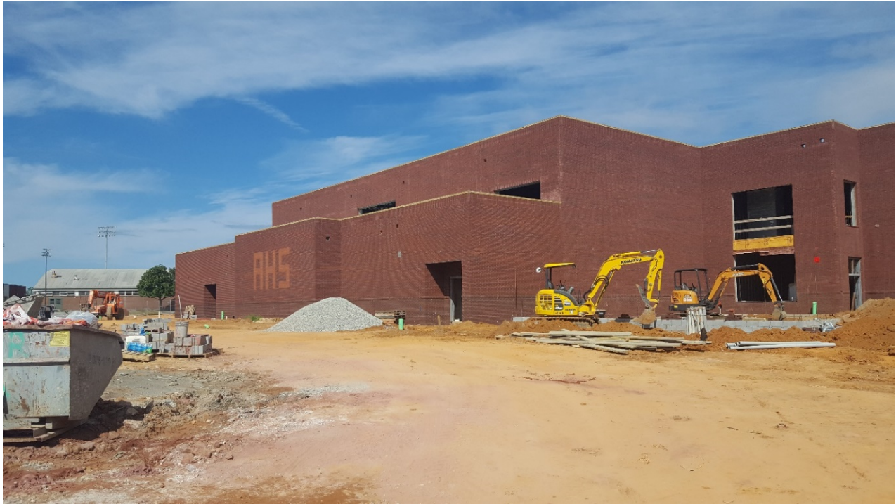
Exterior brick veneer complete south side of Gym Building. Utility work underway at equipment yard.
