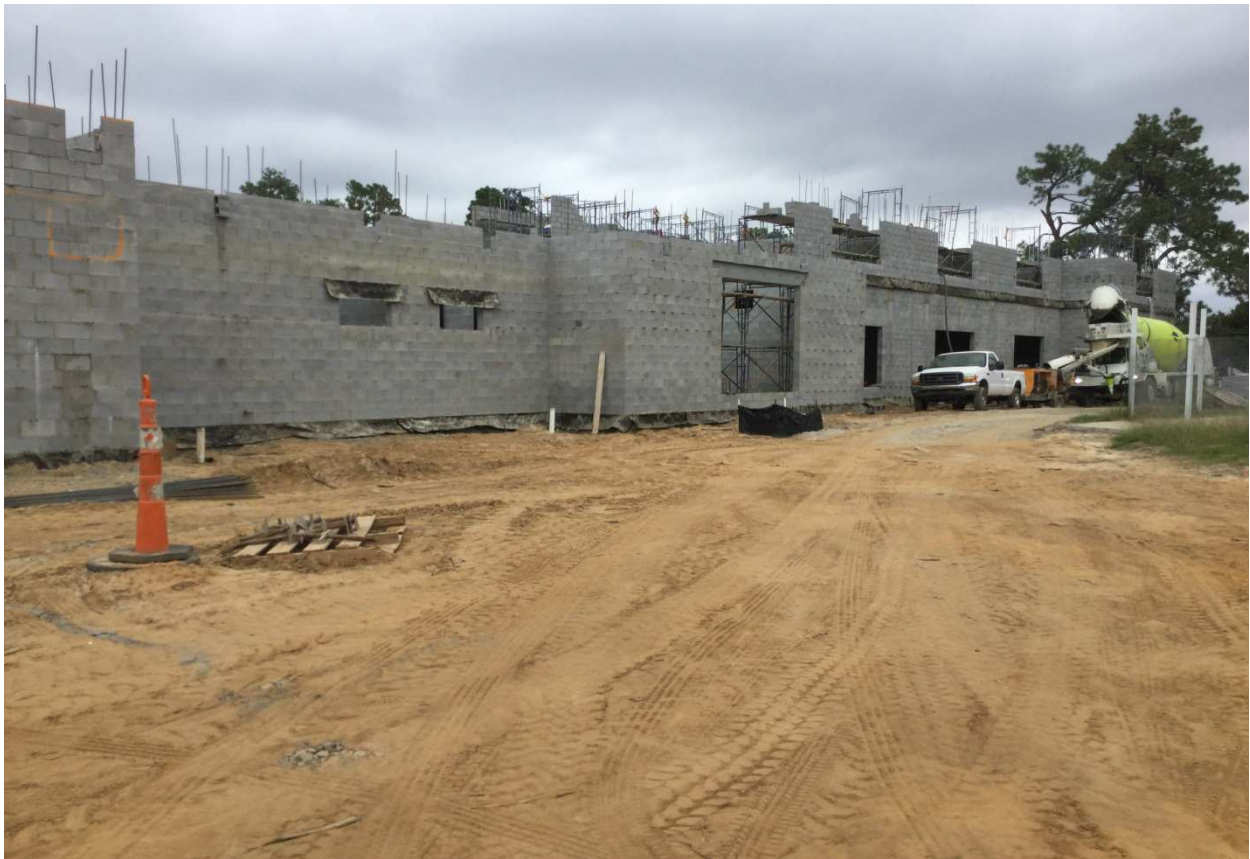
2 nd floor CMU walls underway at area A
