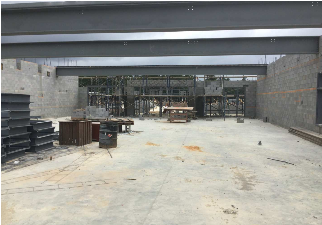
Structural steel at Media center (area B)
