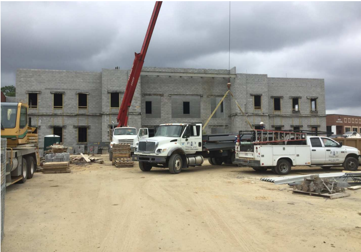
Setting stairs for Admin Building
