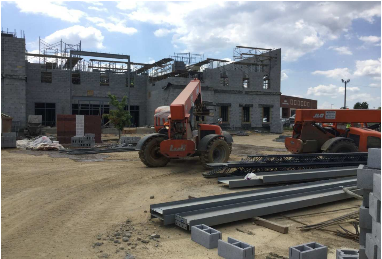
Main entrance and 2 nd floor CMU walls at area E
