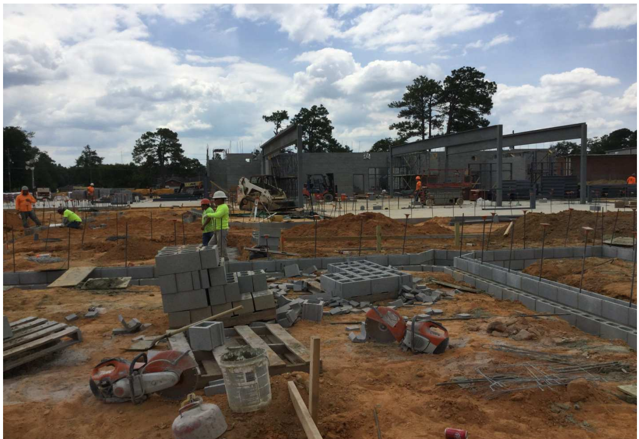
Foundation walls in progress at Area B tie in to new C wing
