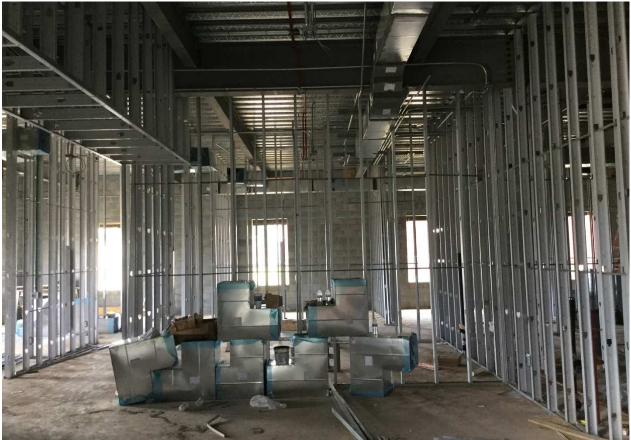
Interior stud framing and overhead MEP rough in at Admin Building (area E)
