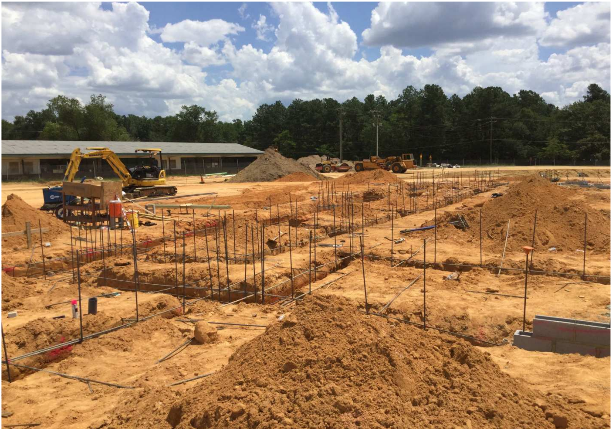
Footing and Rebar Installation at Areas A & B
