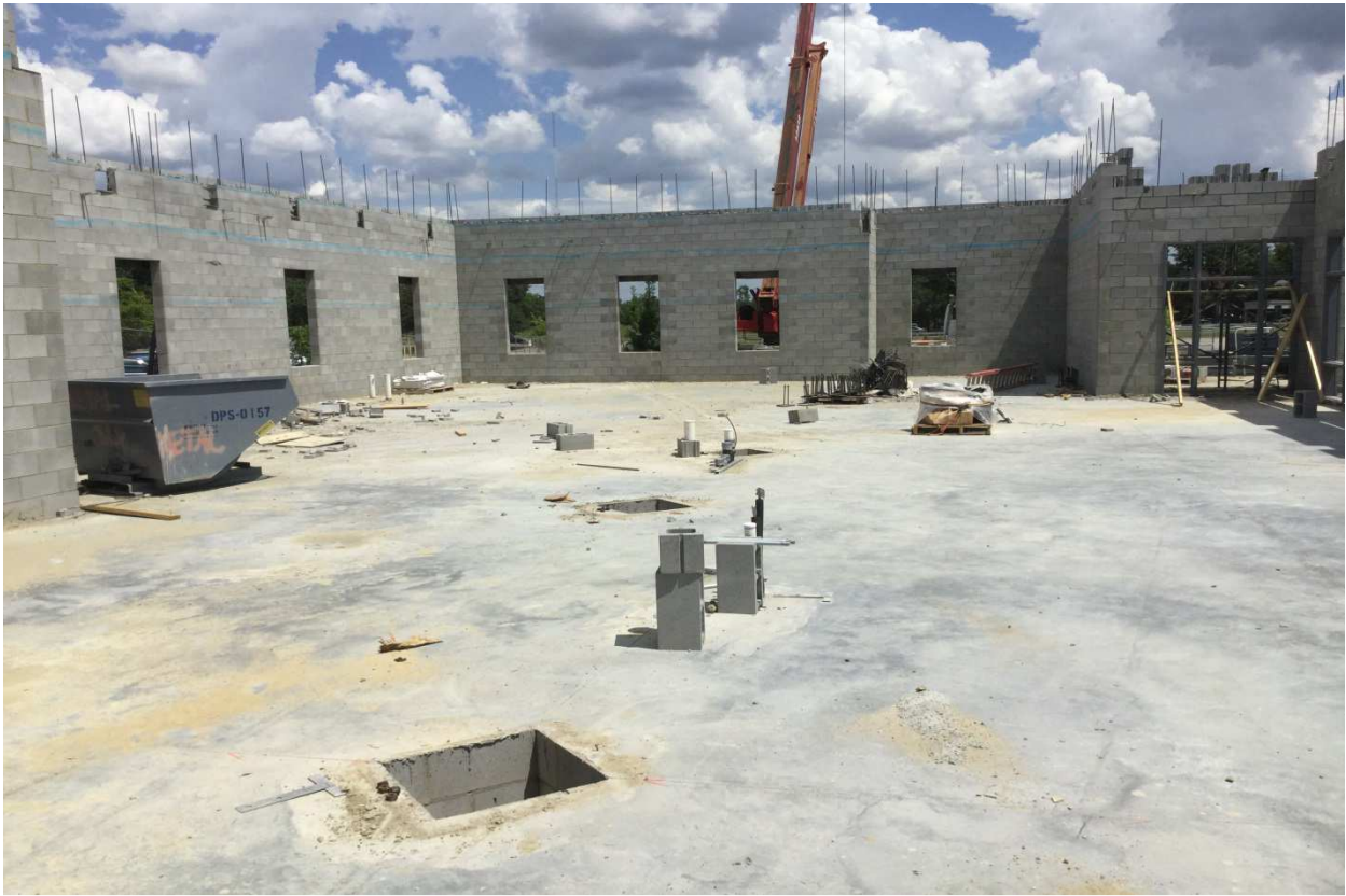
Admin Area Walls
