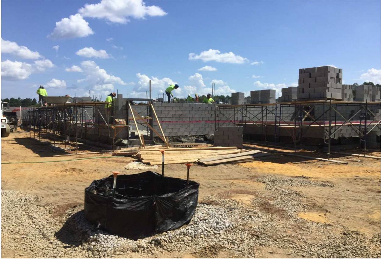
Blockwork underway at Area C
