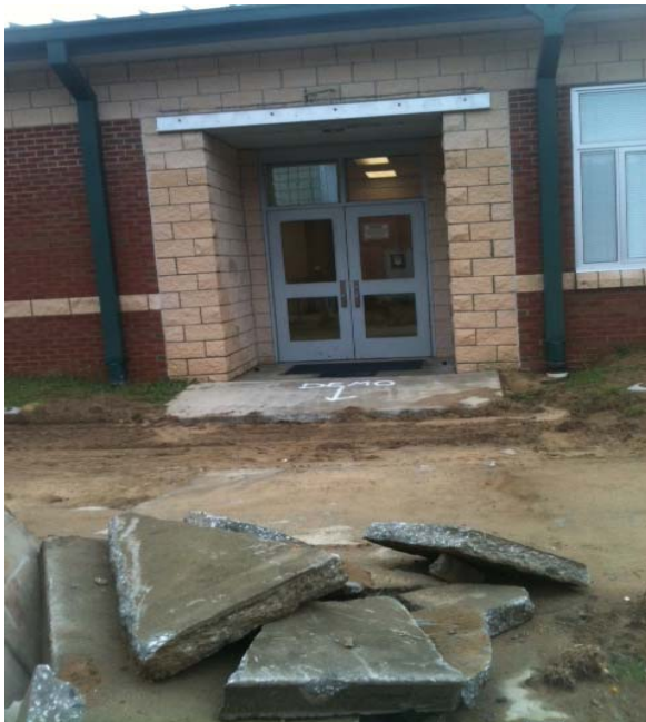
3- Site demolition at connection to existing building.
