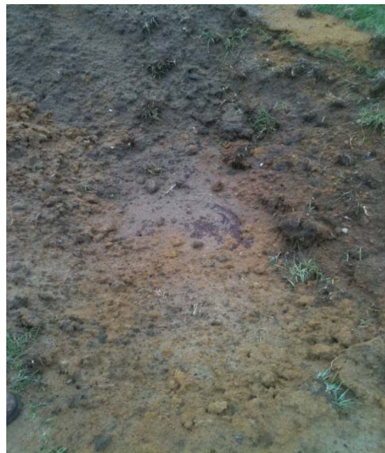
4- Unmarked (buried 2' deep) sanitary sewer line discovered.
