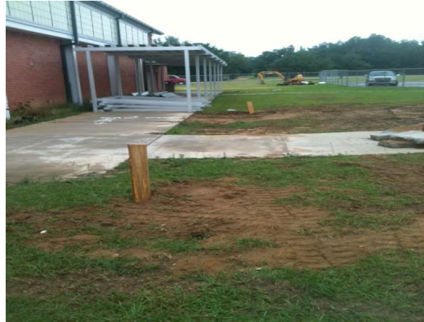
2– Existing walkway cover partially removed.
