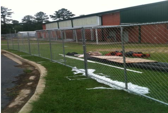
1 – Construction site fencing along car loop.
