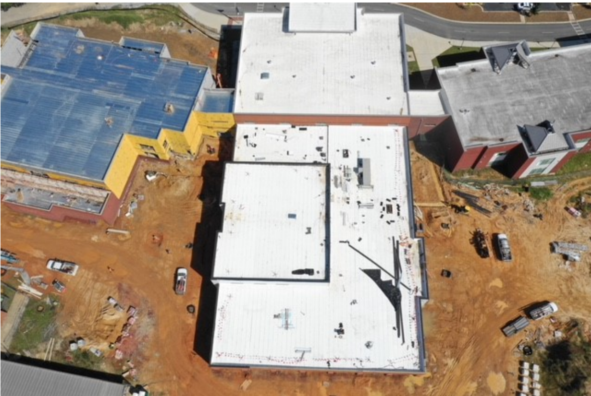
Temporary roof dry in at ROTC/Band building. Steel deck on Gym Building.
