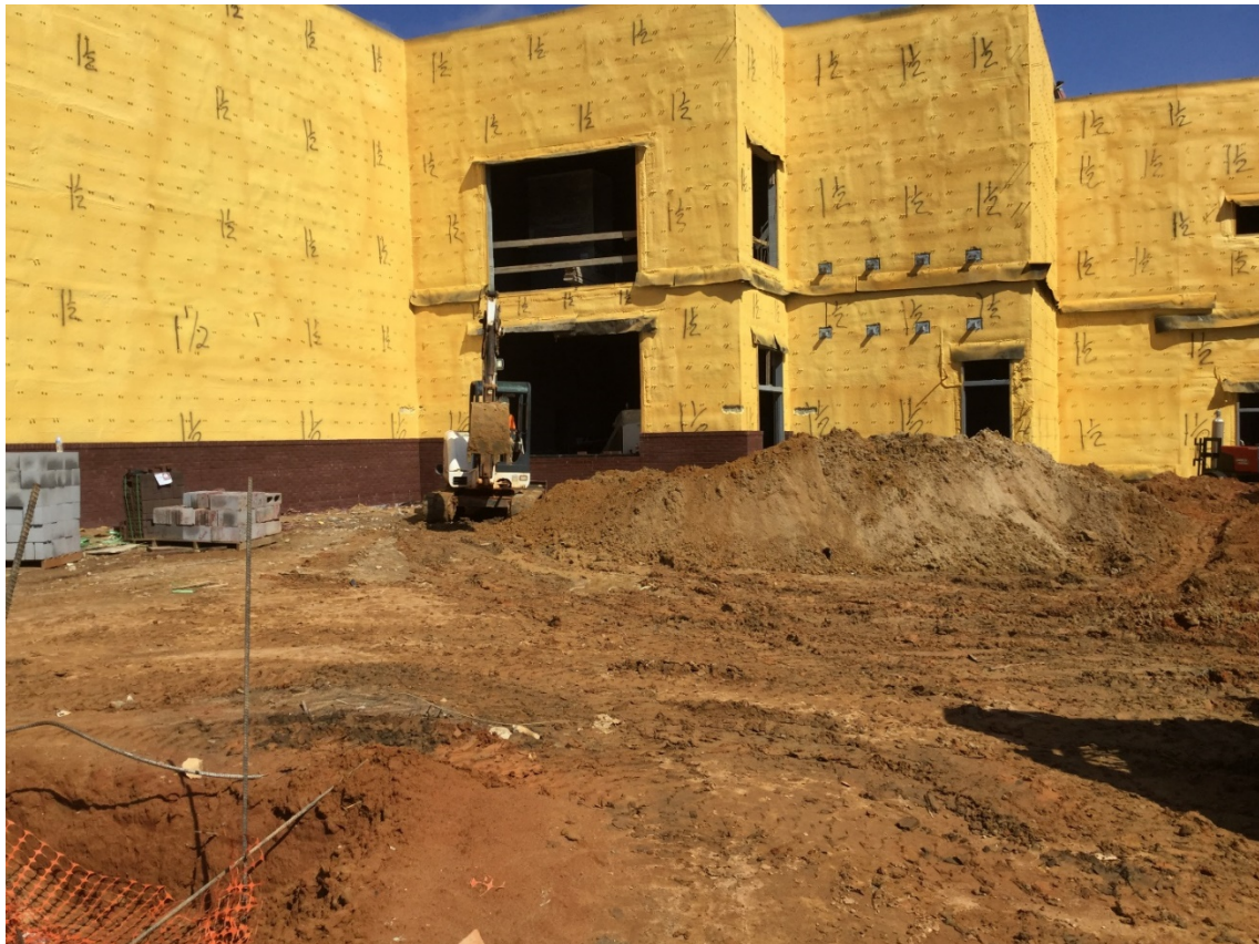
Future mechanical equipment yard. Spray foam insulation complete at Gym building connector.
