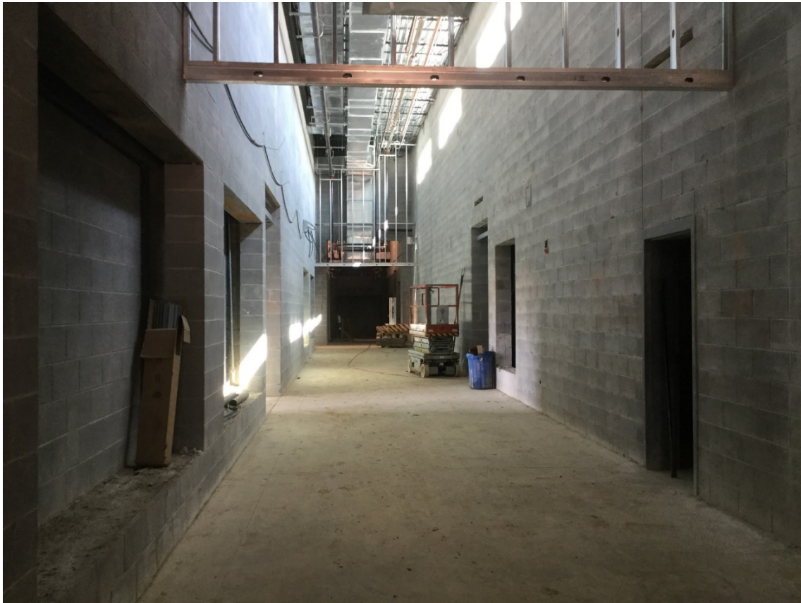
Misc. metal stud framing underway at Band/ROTC building corridor.
