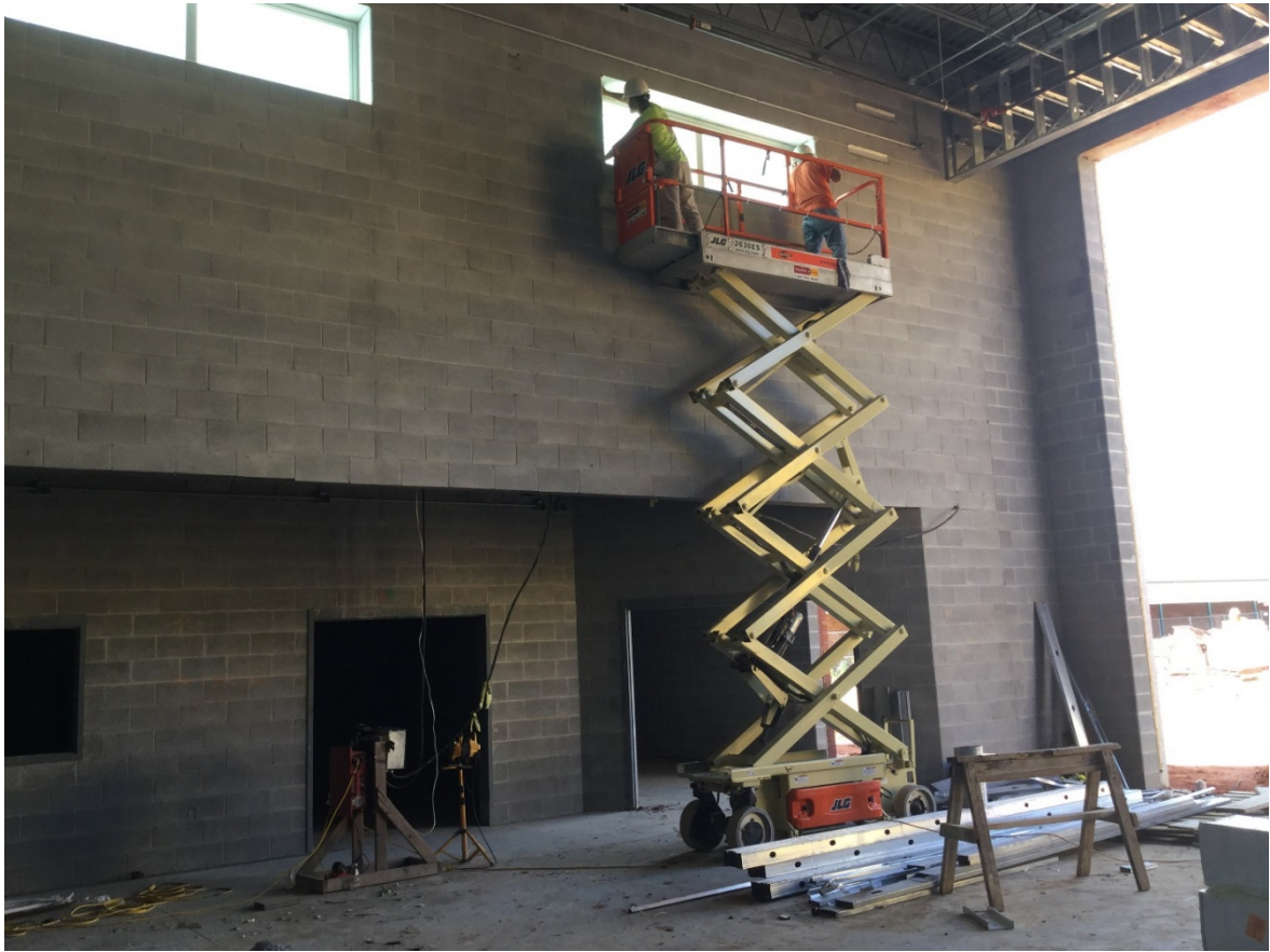
Installation of windows in Band Room.
