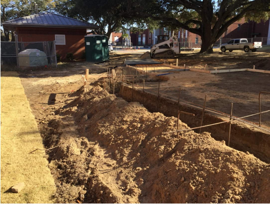
Footers for new retaining wall at outdoor learning area.
