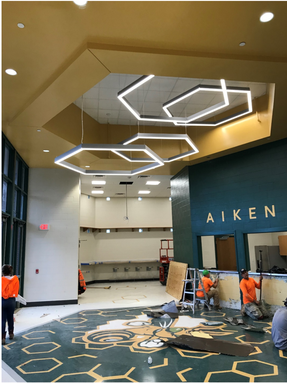
Completing work in lobby.
