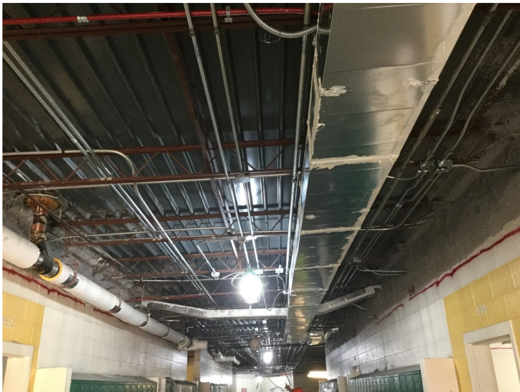
New ductwork installed above ceiling in corridor of classroom wing.
