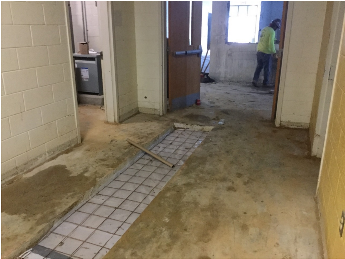
Slab prep for concrete patch at new underslab plumbing rough-ins.
