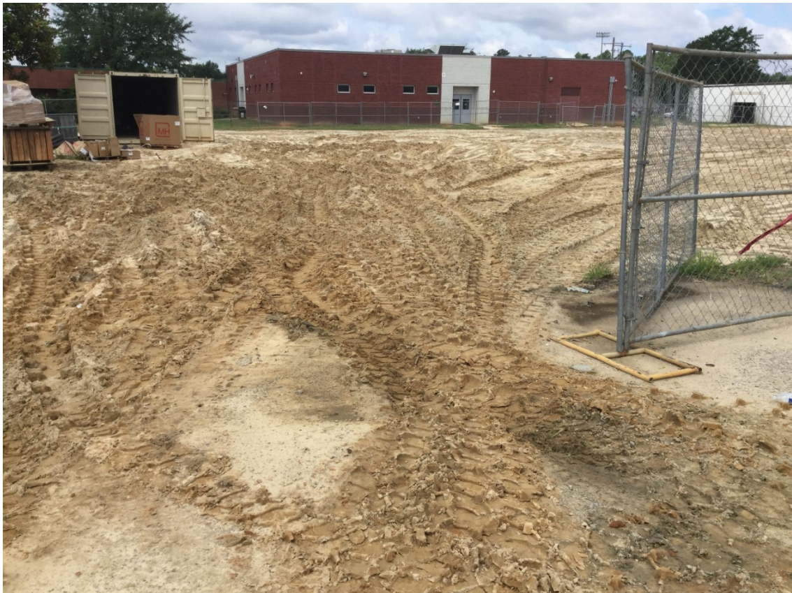
Old Barrel Gym has been removed and is now the designated material storage yard.
