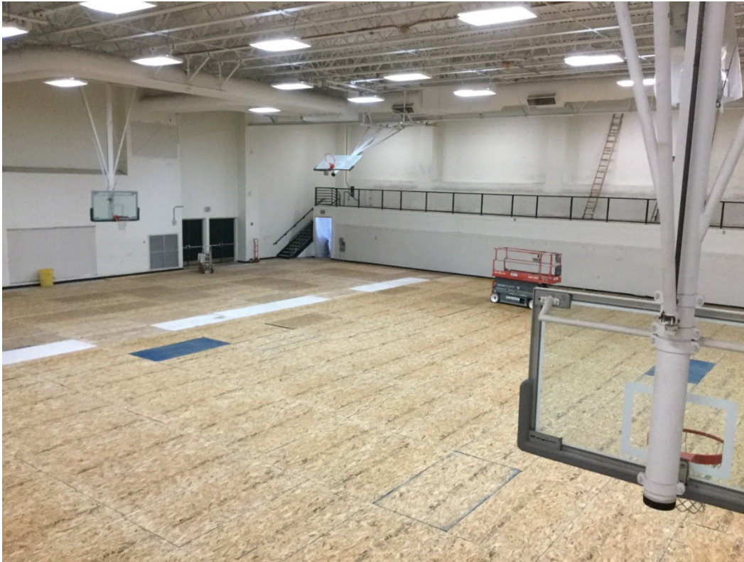
Old bleachers removed. Floor protected while performing new overhead rough-ins.
