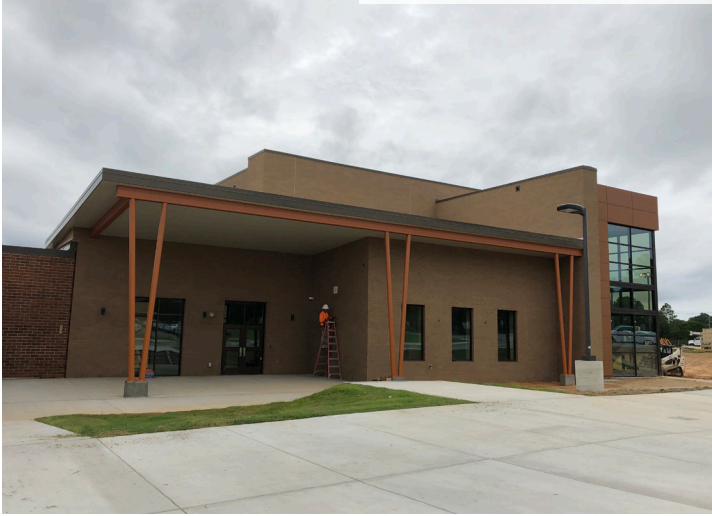
AREA C - NORTH FACADE
