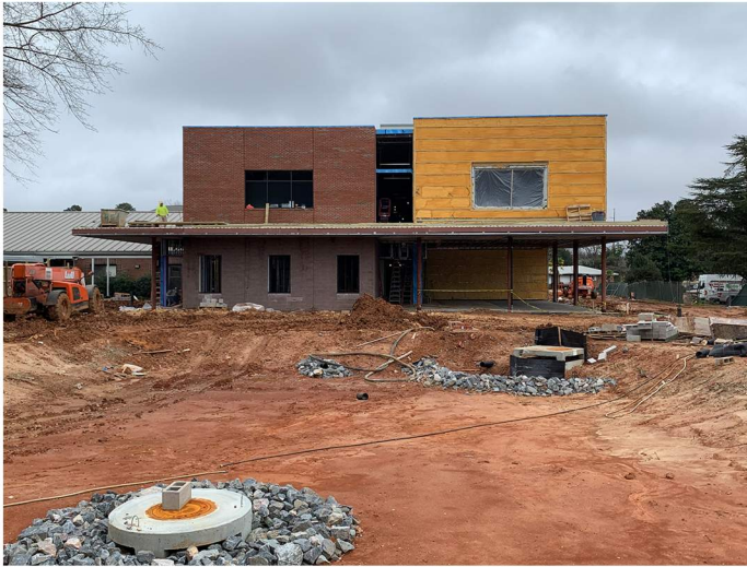
Exterior progress photo.
