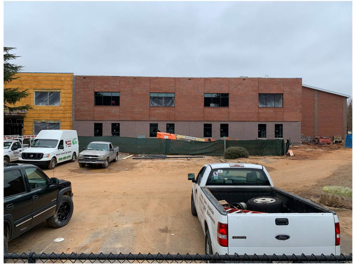
Exterior progress photo.
