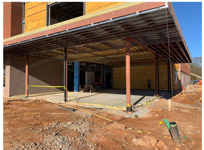
Concrete has been poured for the plaza at the main entry.
