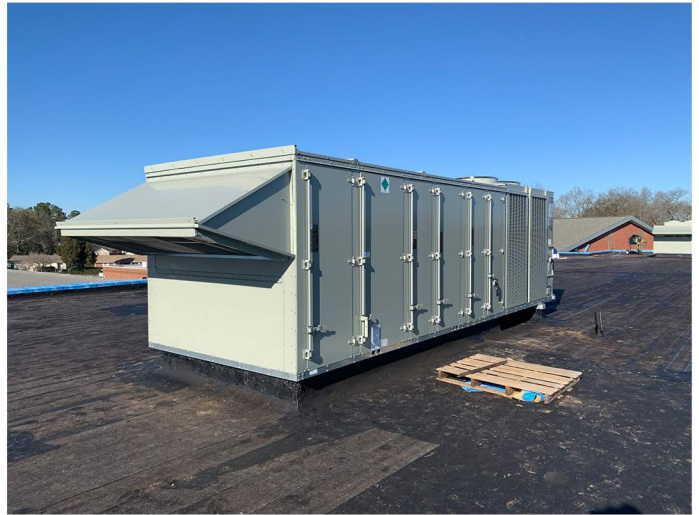
The main roof is dried in and mechanical units are set.
