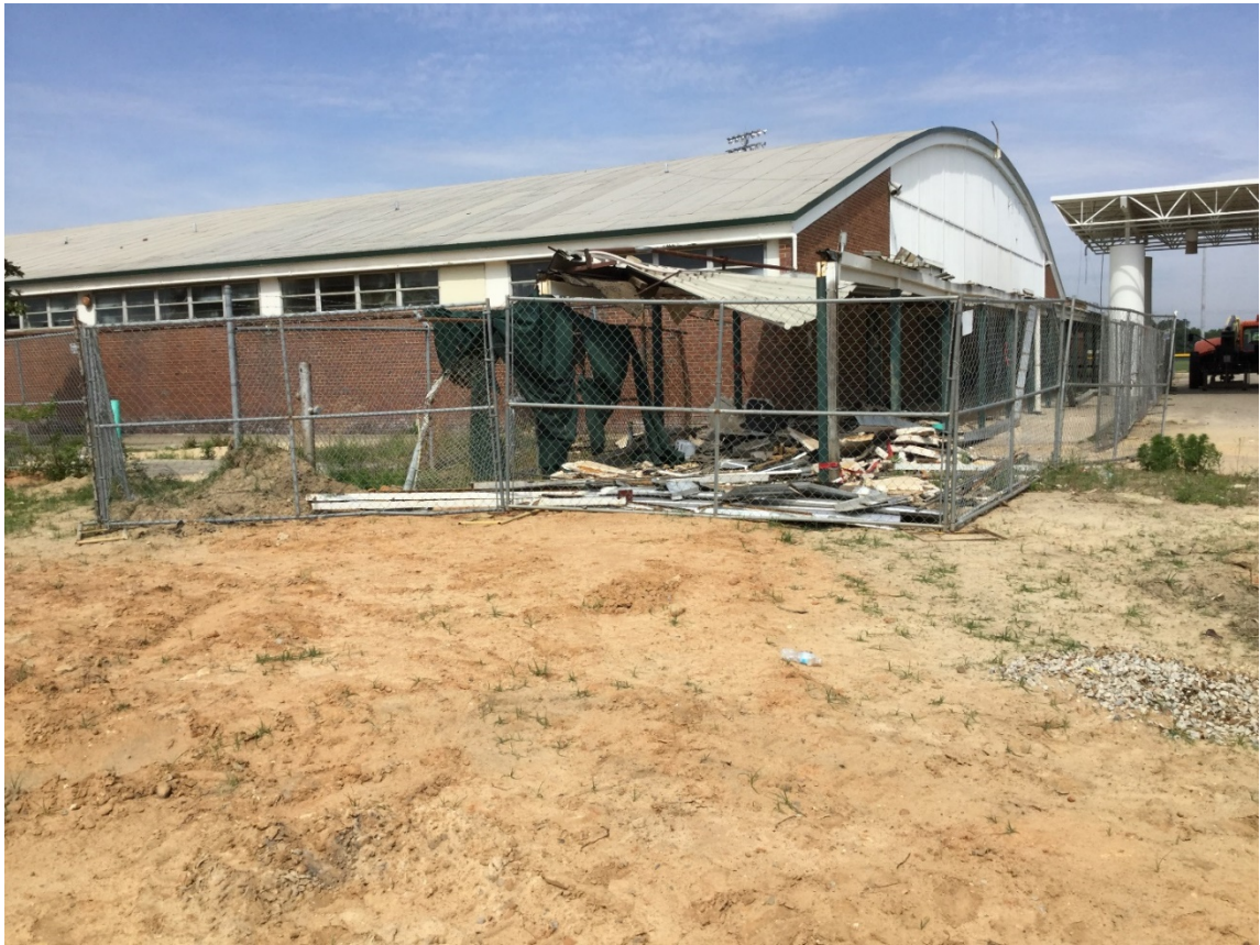
Demolition starting at existing 'Barrell' gym.
