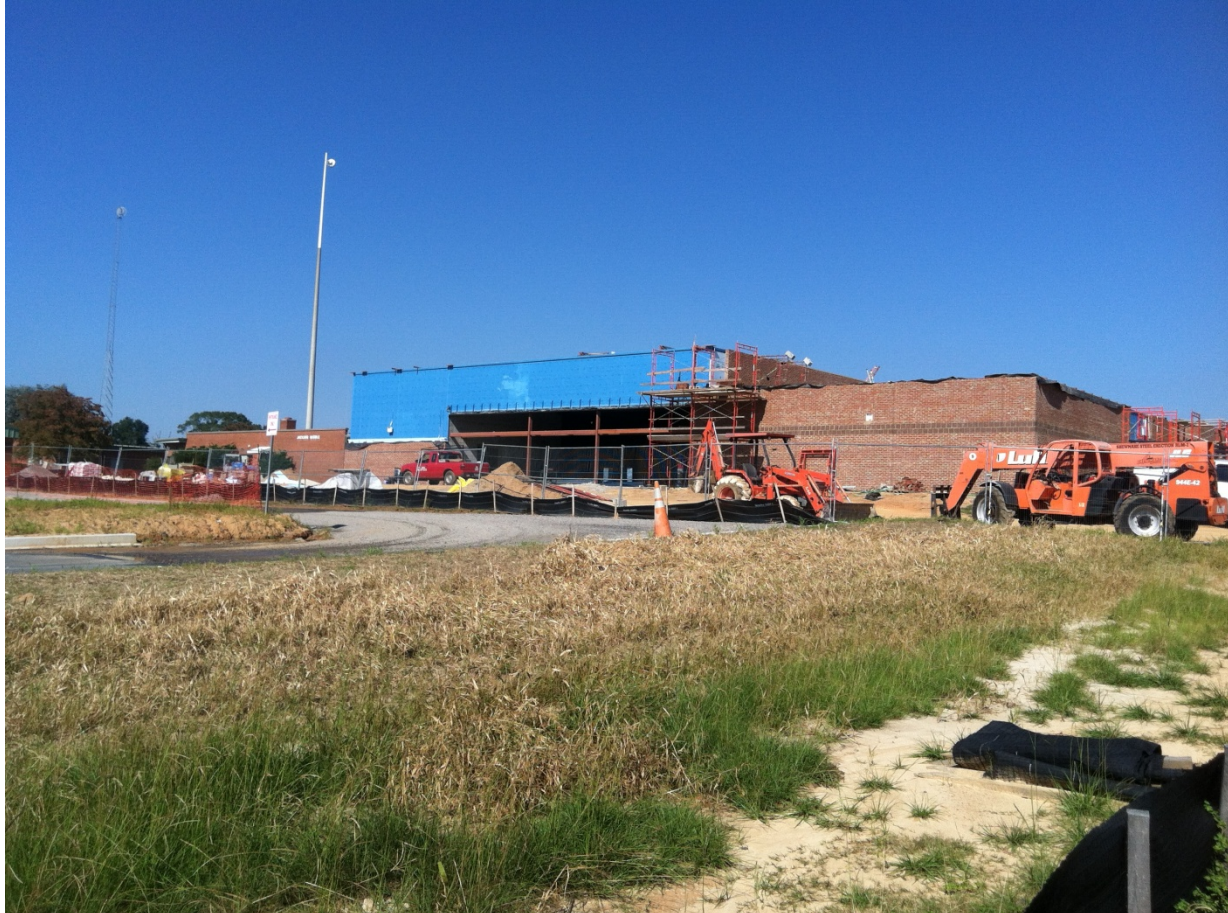
1 – Addition viewed from Atomic Road. Brick veneer is complete above the lower roof areas in advance preparation for roofing.
