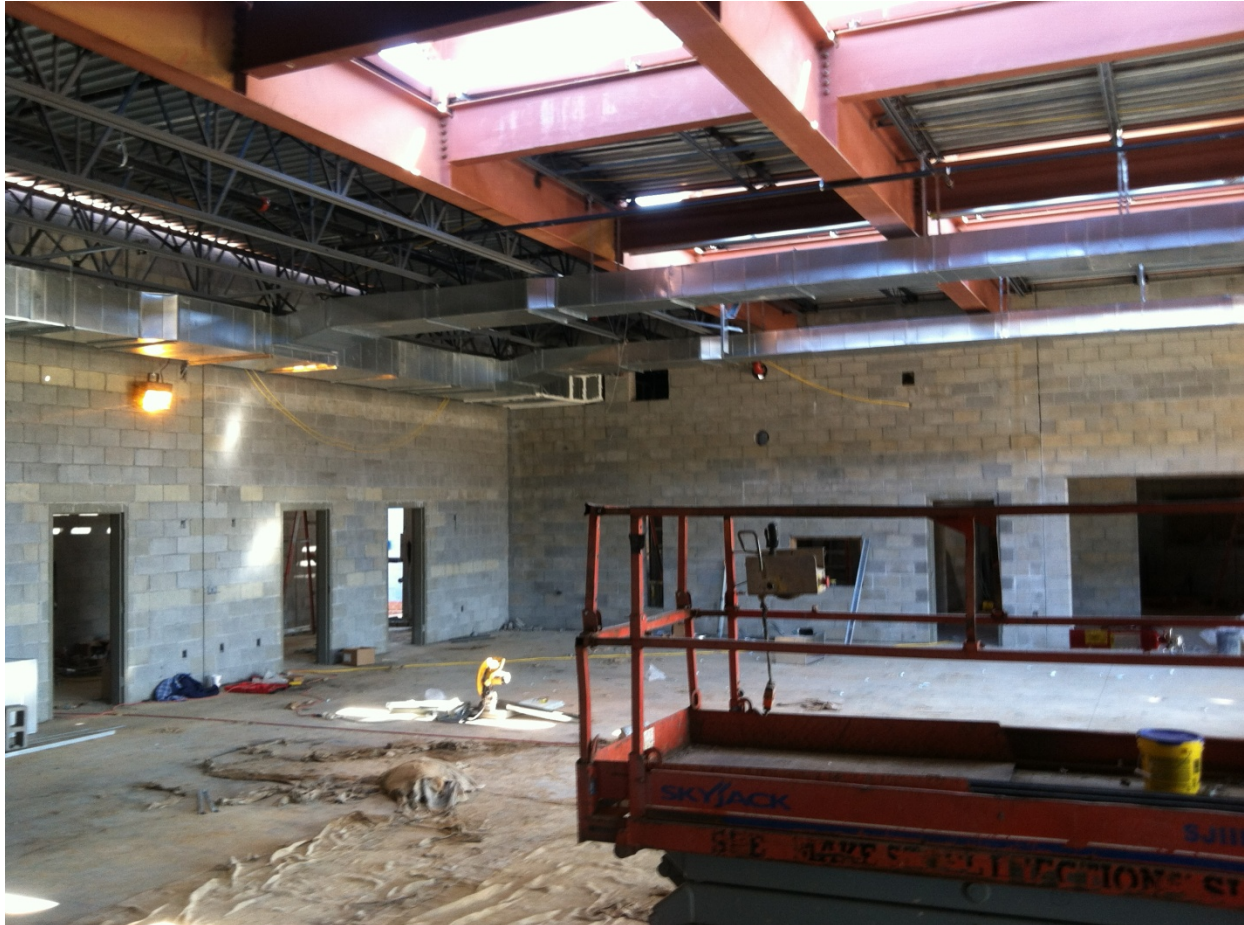
2 – Dining Room interior. Roof monitors admit light deep into the building, as visible in photo. Supplemental construction lighting has not been necessary.
