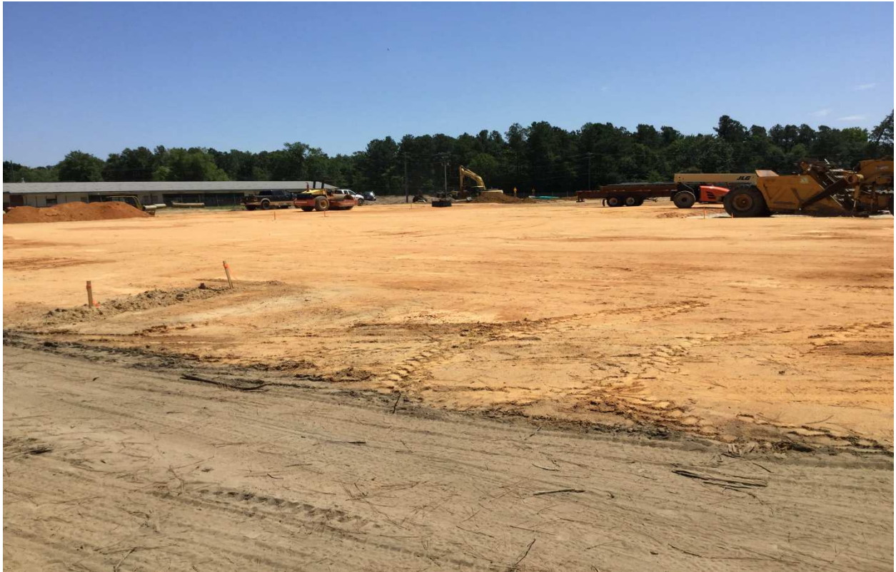
Building pad backfill at Cafeteria
