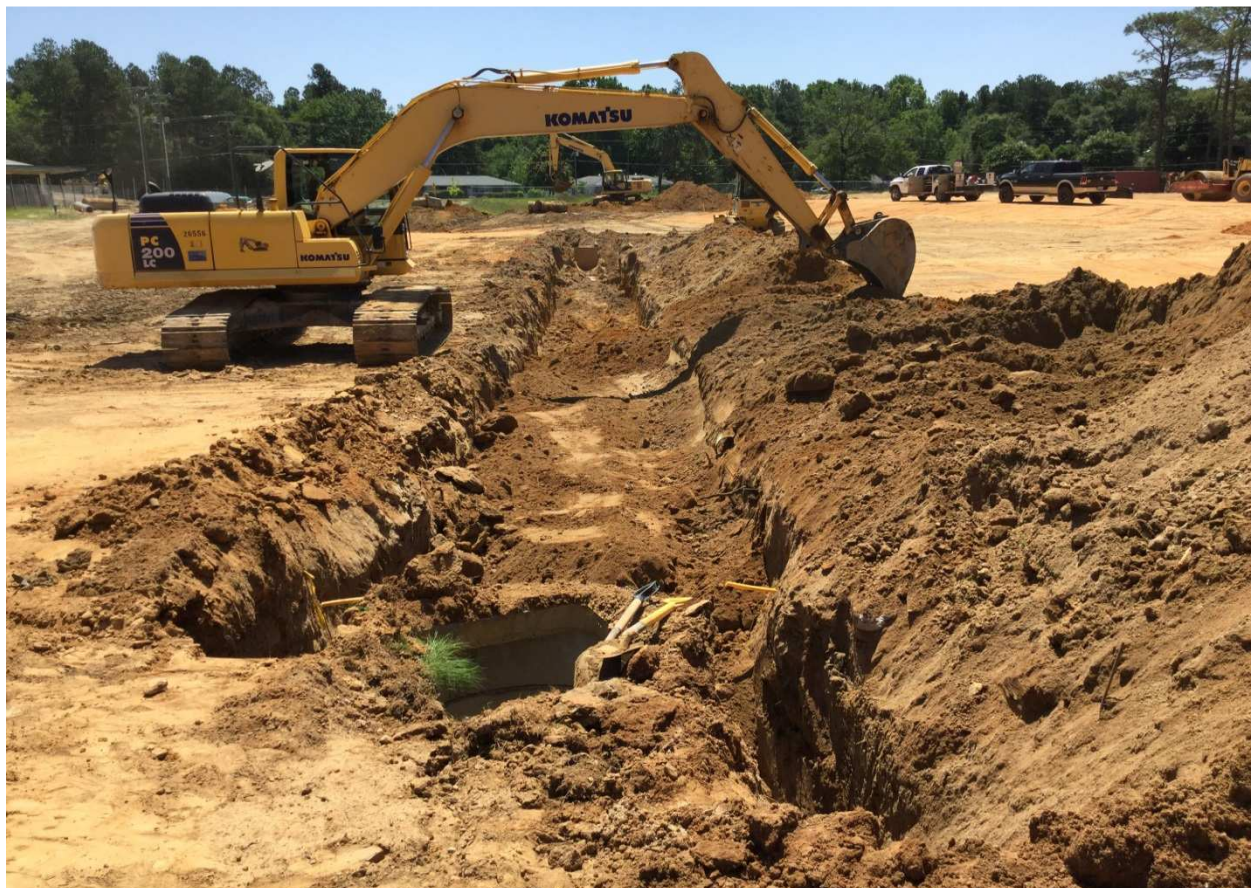
Removal of existing storm drain Area D
