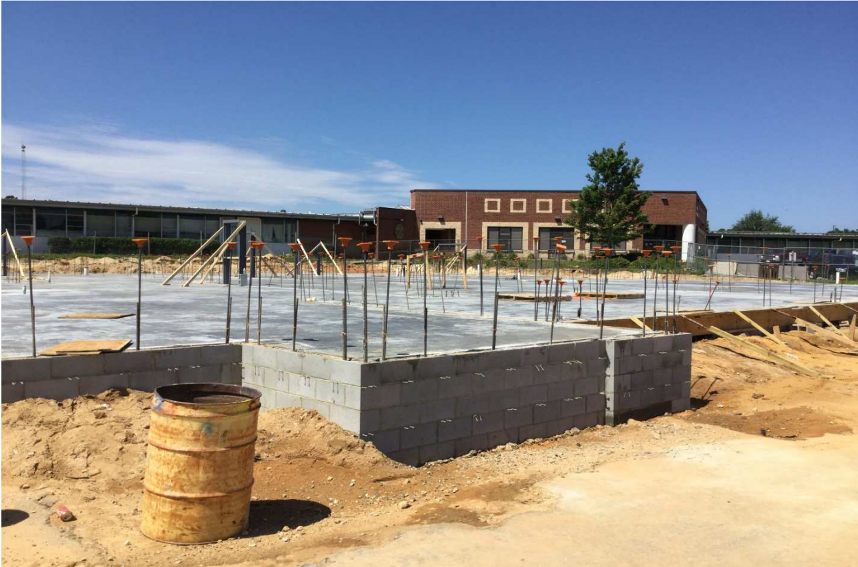
Foundation wall and slab on grade Admin Building
