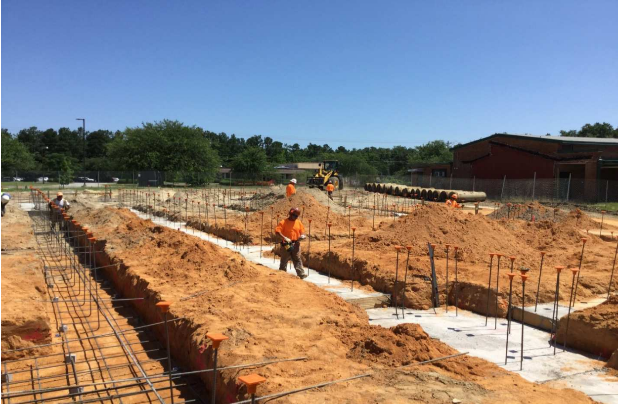
Footers in progress at Area C
