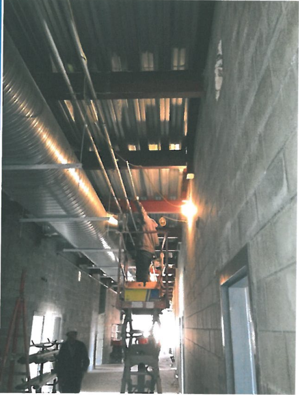
Science Building Ductwork & Electrical
