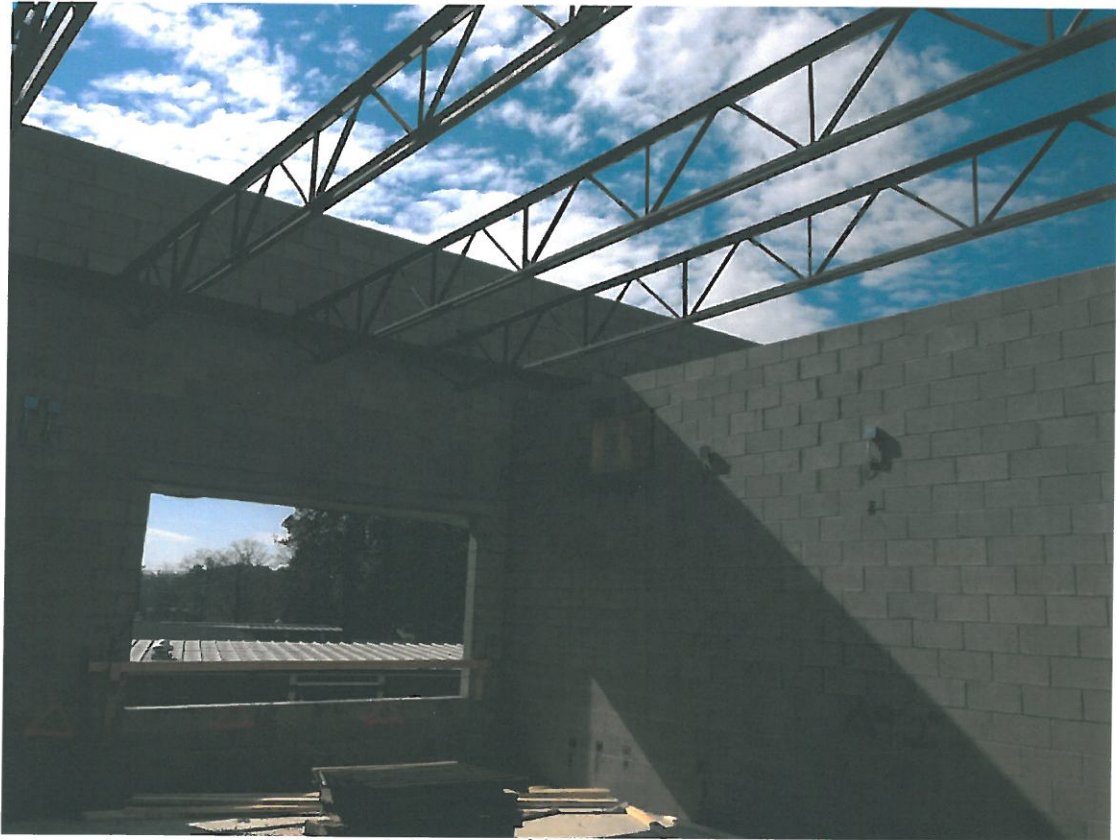
Science Building Roof Joists
