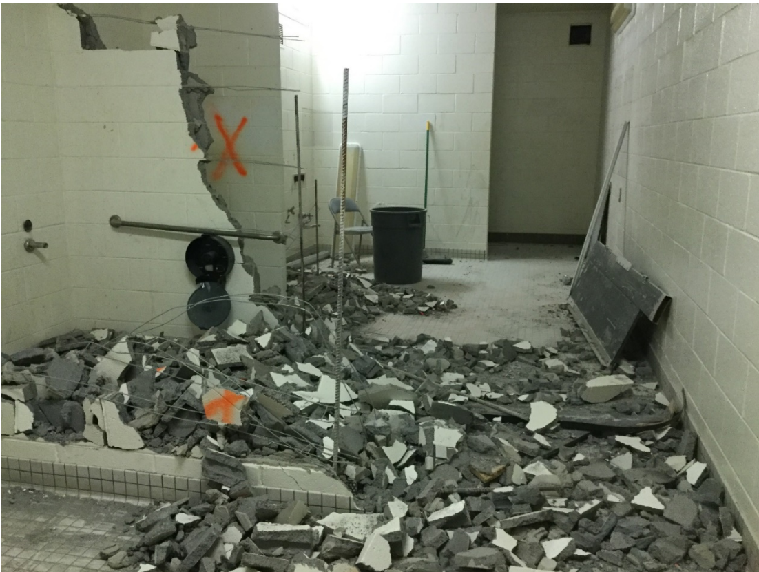
Demolition of walls and floors at existing locker rooms.
