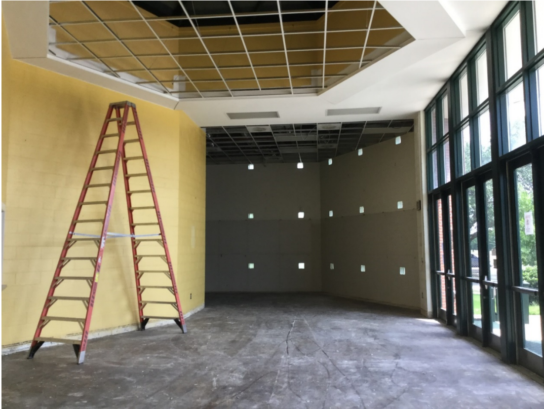
Existing finishes removed at front lobby.
