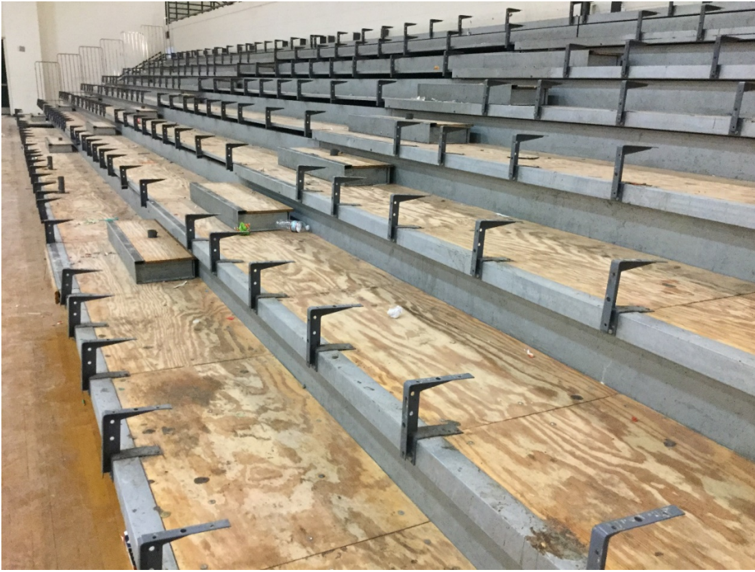
Removal of bleachers underway.
