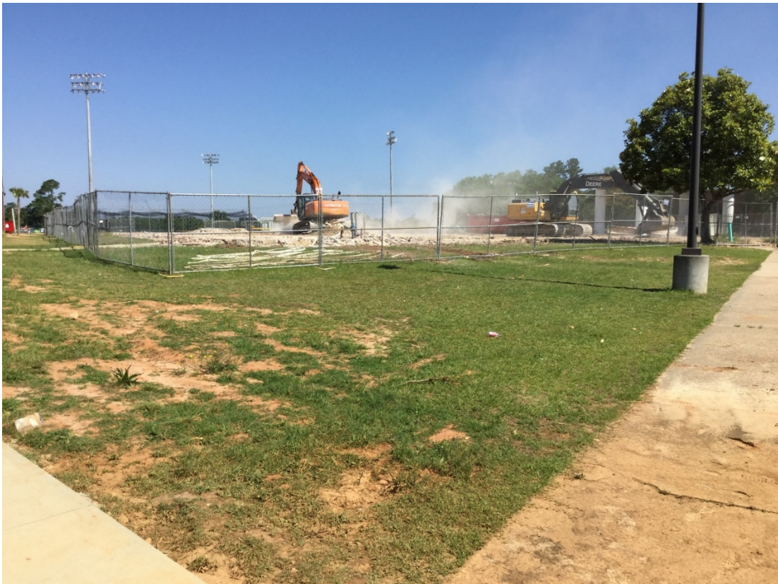
Removal of old Barrell Gym as part of remaining scope of Phase 2B project.
