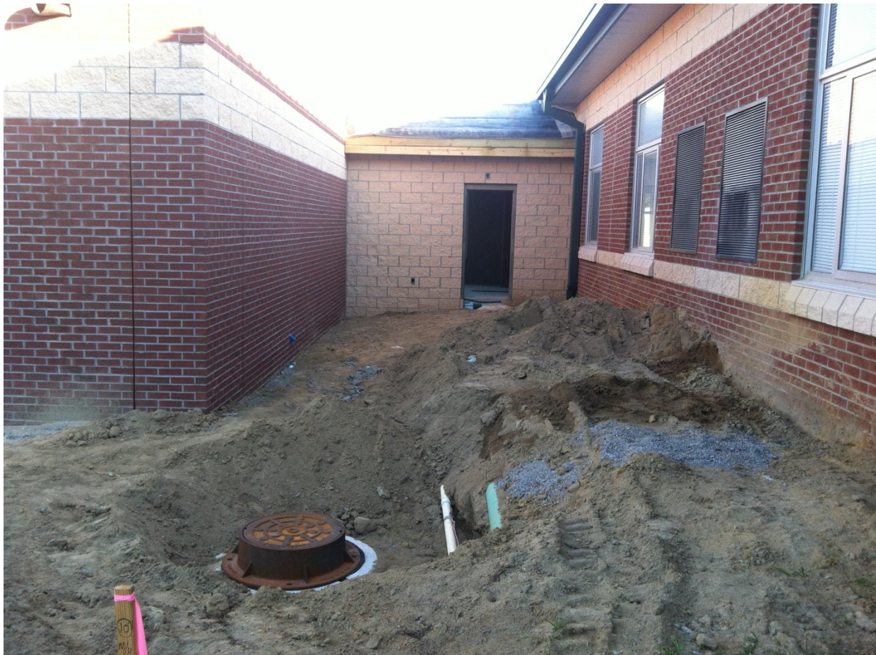
2- Addition from the south. Masonry veneer has been cleaned. Sewer manhole is part of the system from the gym that was re-routed or replaced.
