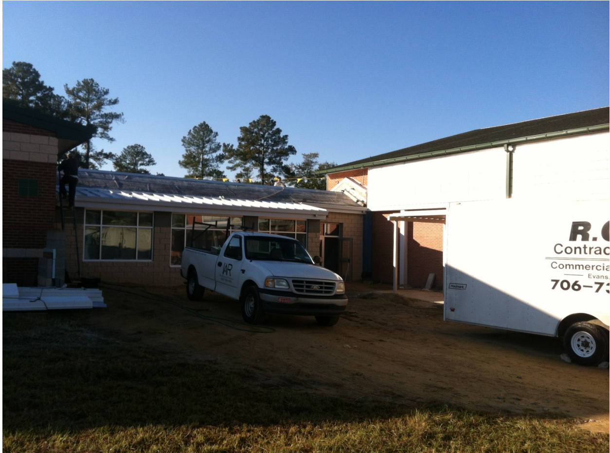
1 – Addition viewed from the north. Glass is installed, and the metal roofing is started.
