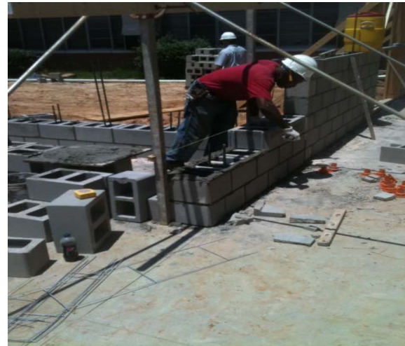
4- Masons at work on 12" cmu firewall.
