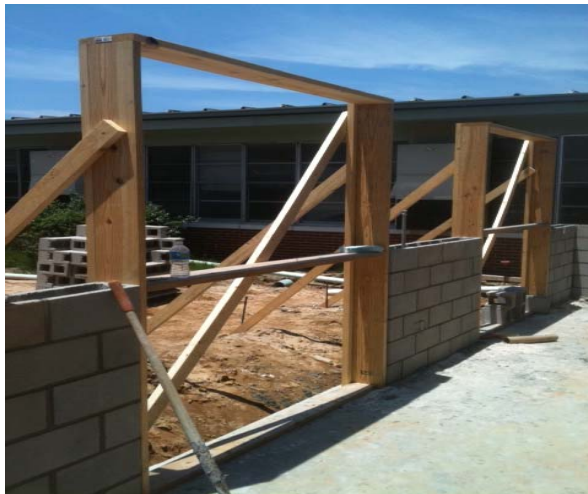
3- Masonry openings are blocked-out for curtain wall to be installed later.
