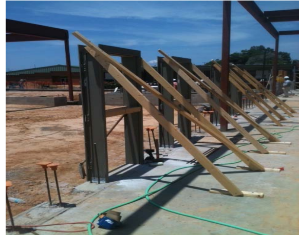
2– Door frames set along corridor, ready for CMU wall construction. Structural steel frame is partially set.
