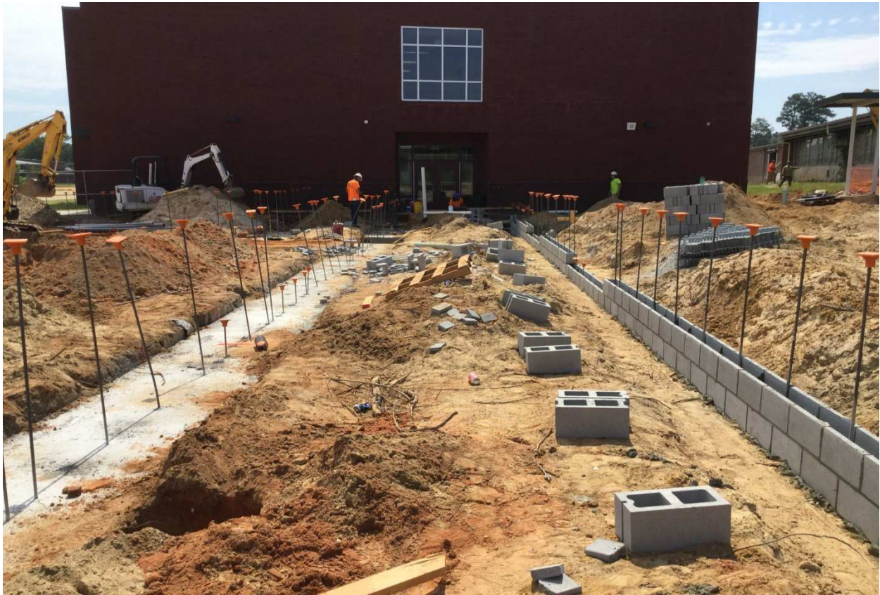
Foundations of Admin Building underway
