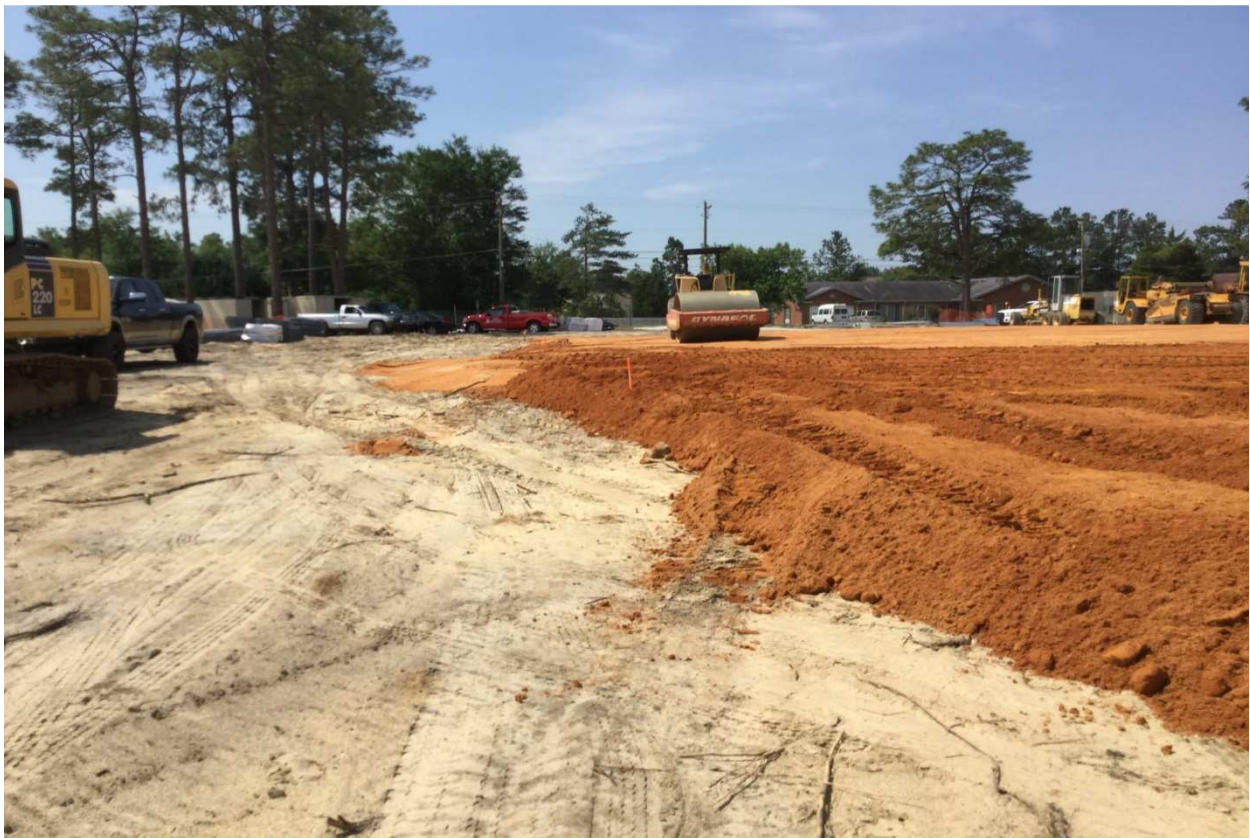
Building pad grading at new classroom addition
