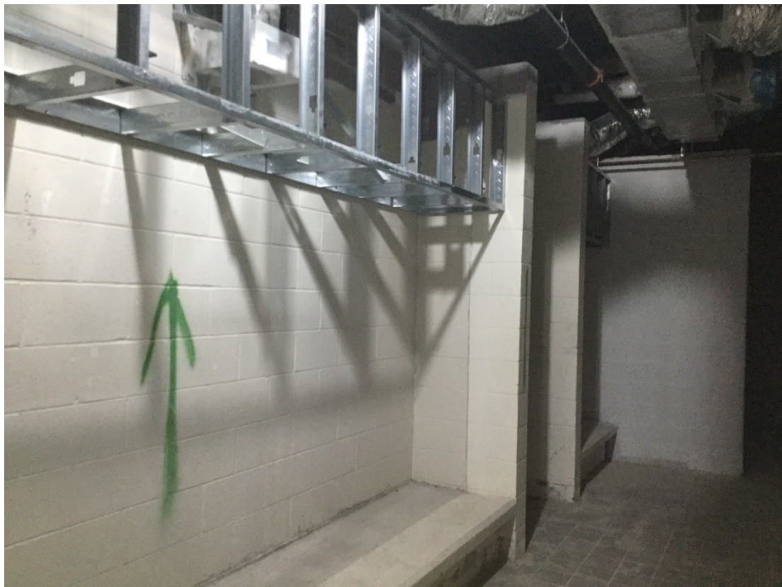
Framing gypsum soffits and ceilings.
