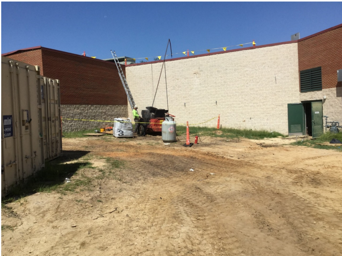
New roof in progress.
