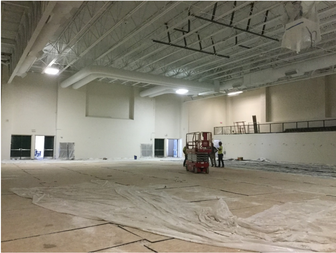
Repainting gym ceiling and ductwork.
