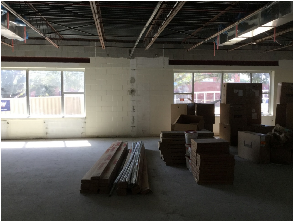
Rough-ins complete at classroom. Stored material for acoustical ceilings and gypsum walls.
