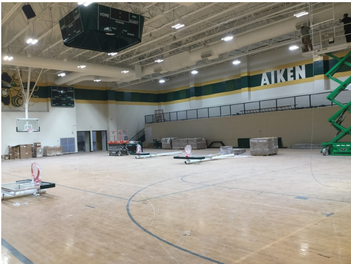
Scoreboard and goals installation completing at gym.
