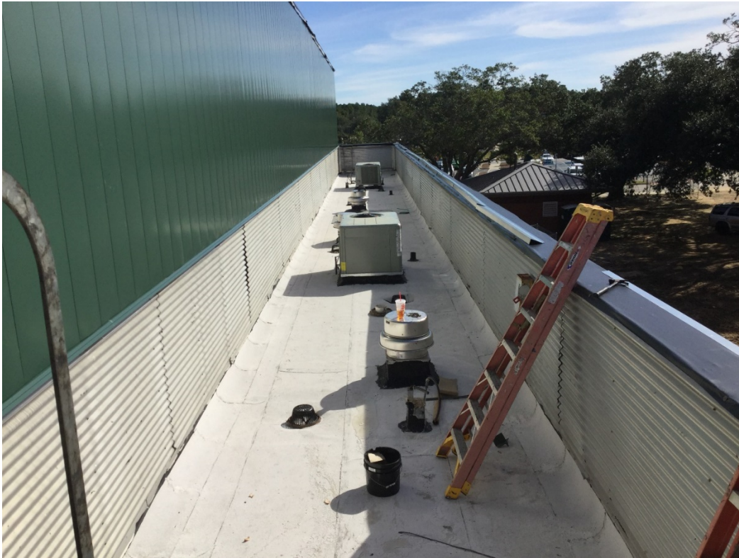
Metal panel installation at roof.
