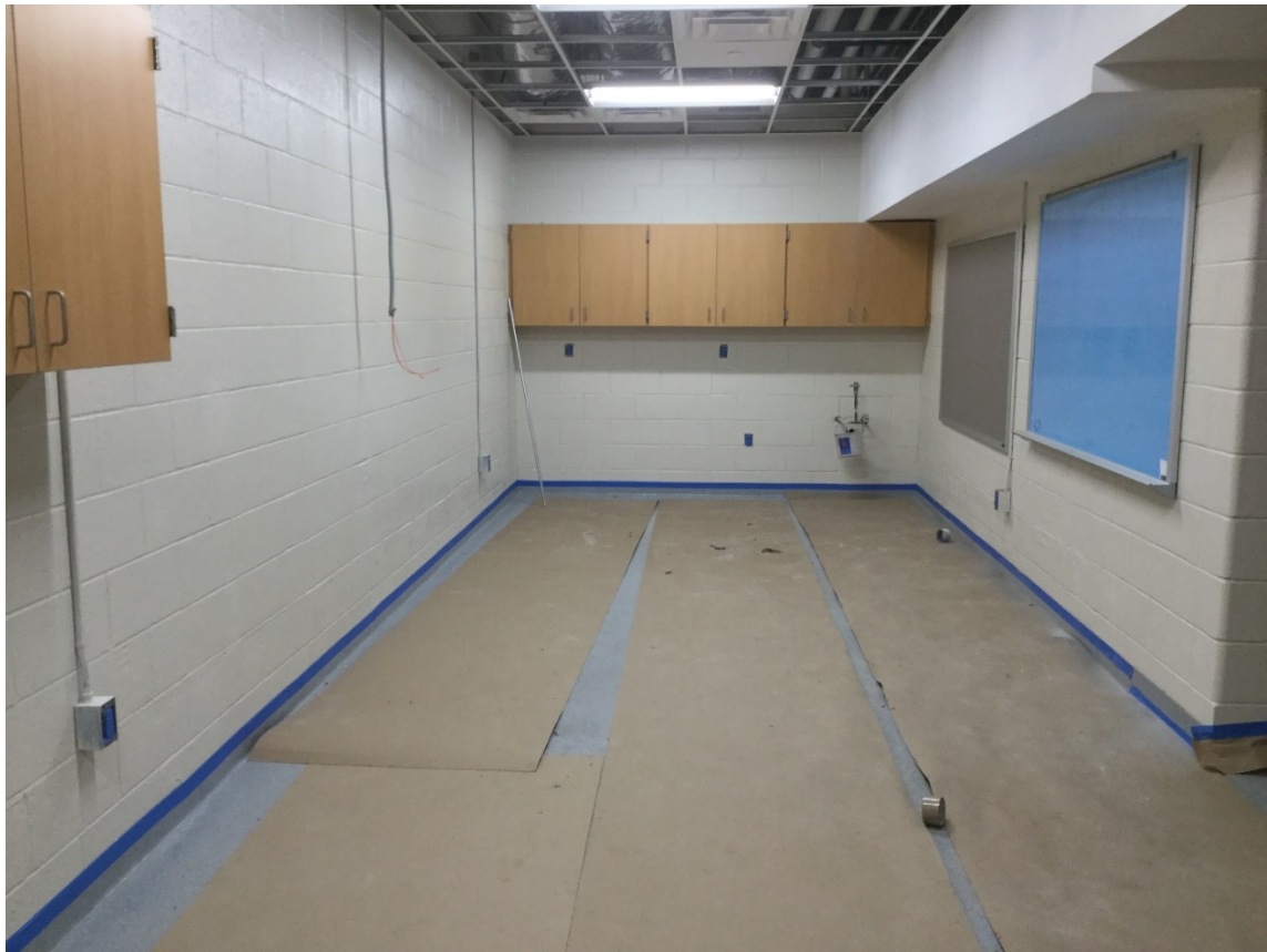
Epoxy flooring, lighting and cabinets installed at new training room.
