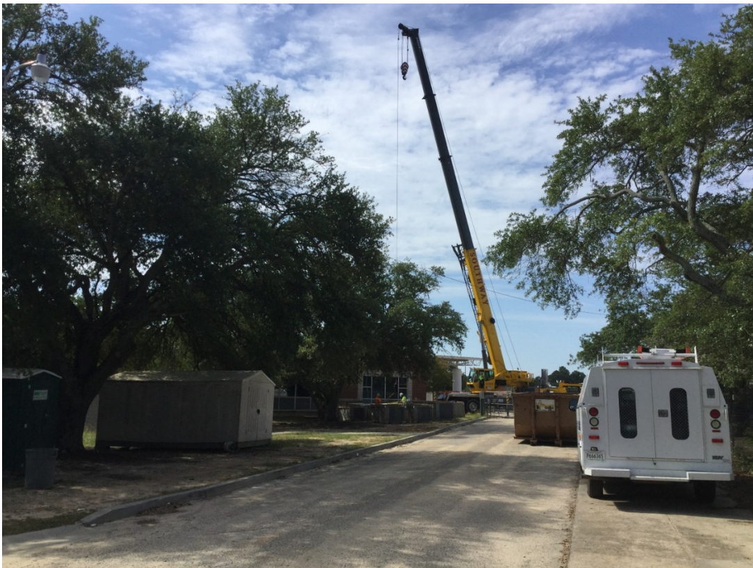
Setting some roof top mechanical units underway
