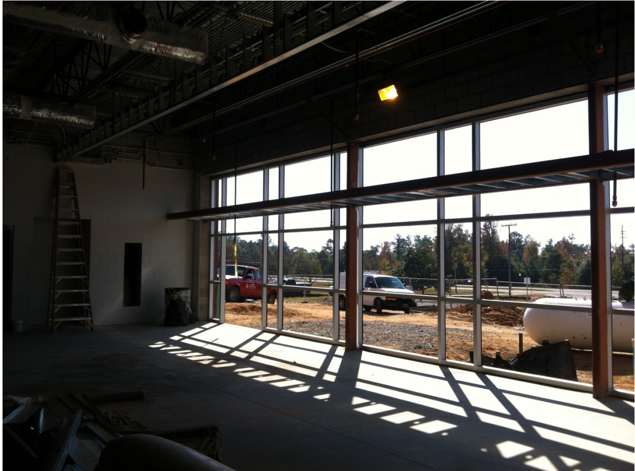
2 – Dining Room interior. Aluminum curtain wall framing is installed. Interior portion of a light shelf has been framed. This will help to reflect natural light into the space.
