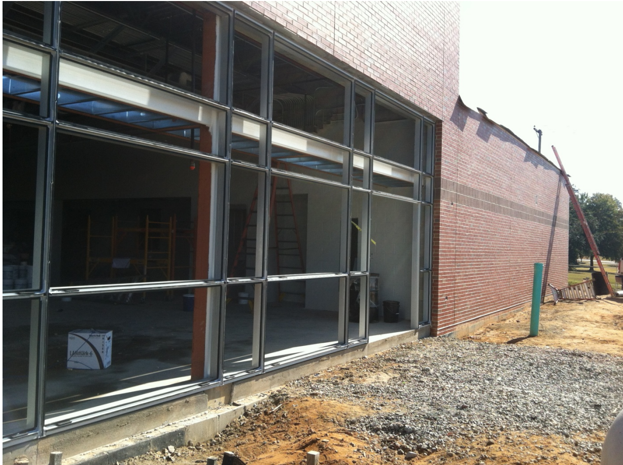
1 – Addition viewed from Atomic Road. Brick veneer is complete and has been cleaned. Aluminum curtain wall framing is in progress.
