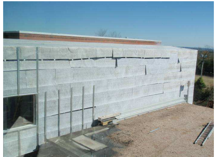
Connecting corridor exterior sheathing and preparation for siding/roof
