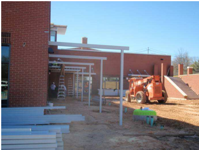
Exterior canopy installation
