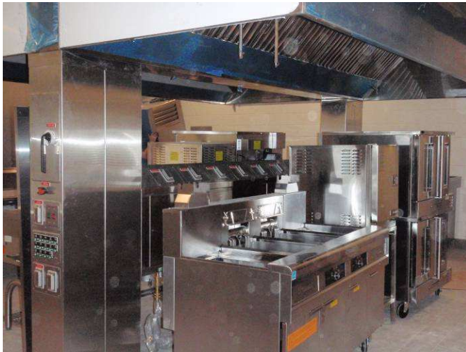
Kitchen equipment installation
