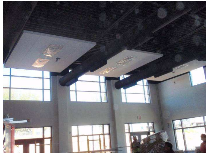
Ceiling installation in Cafeteria
