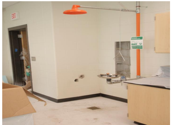
Installing eyewash/shower in Science Lab
