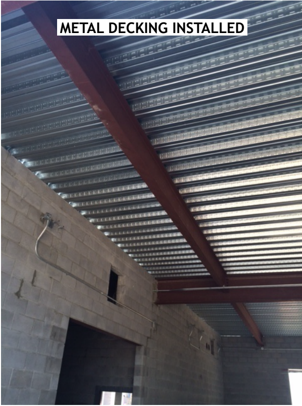
PREP FOR ELEVATED SLAB AREA C
