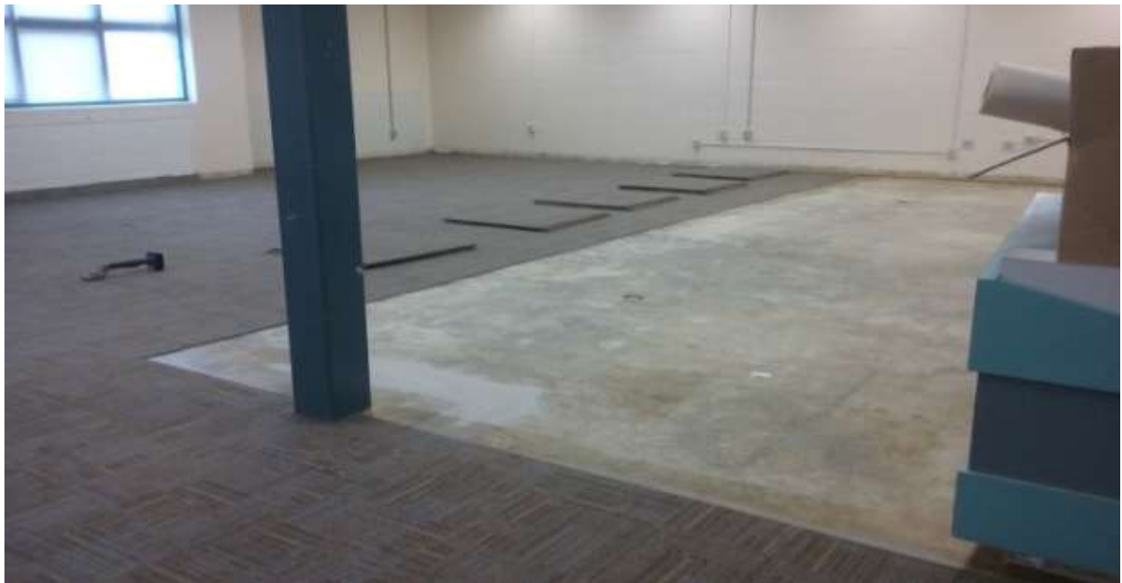
CARPET TILES INSTALLATION @ MEDIA
