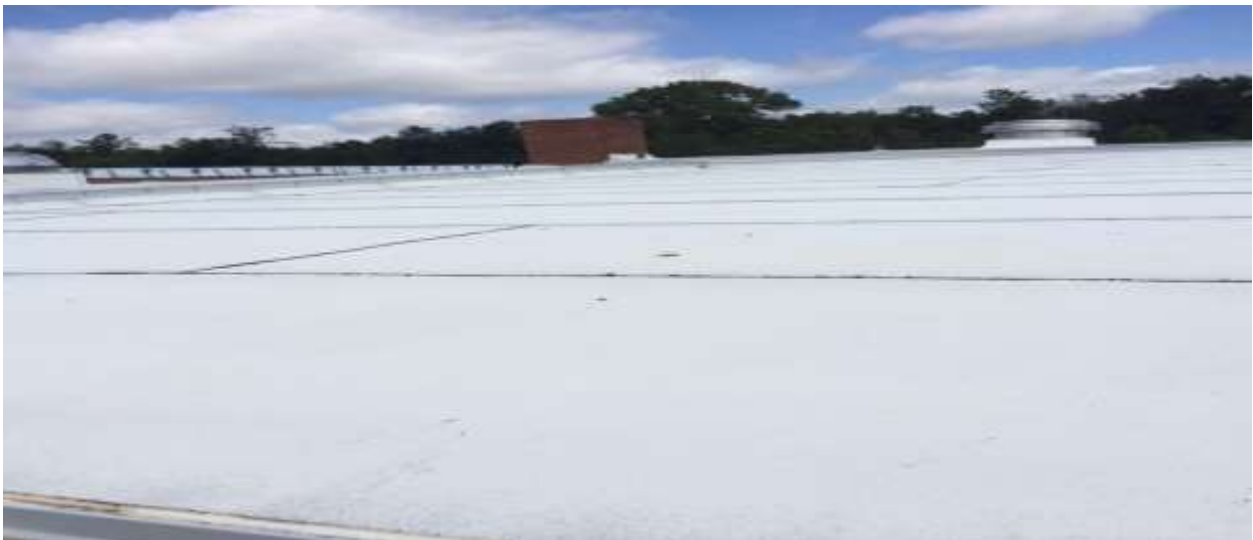
BUILT UP ROOF
