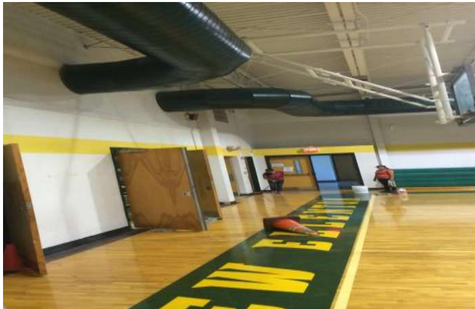
FINISHED PAINTED DUCT AND ACCENT BAND
